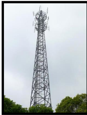
Gambar 9. 8 Sluran Latice tower
